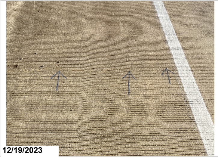
Deck cracking in various locations of deck
