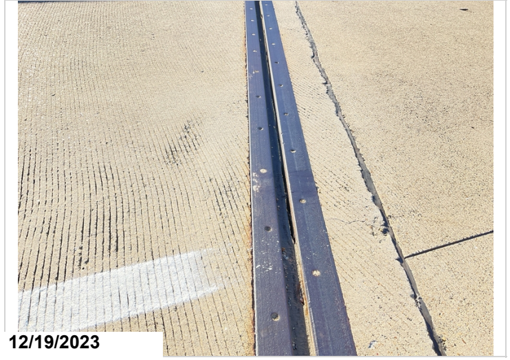
6' of seal damage at end of bridge joint
