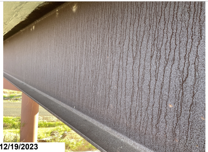
Weathering steel is in good condition
