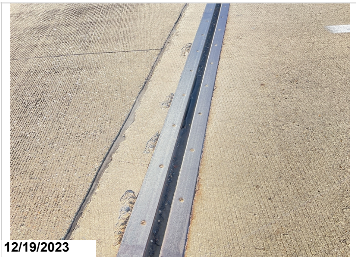
3' of joint material damage at beginning of bridge
