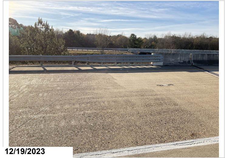
Transition railing, beginning of bridge
