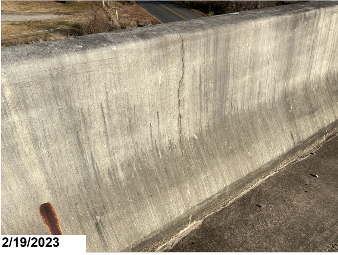
Cracking in bridge railing
