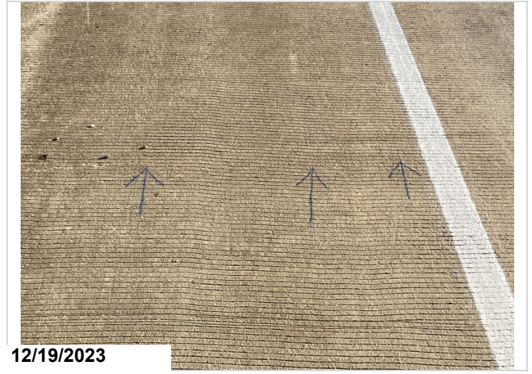
Deck cracking in various locations of deck
