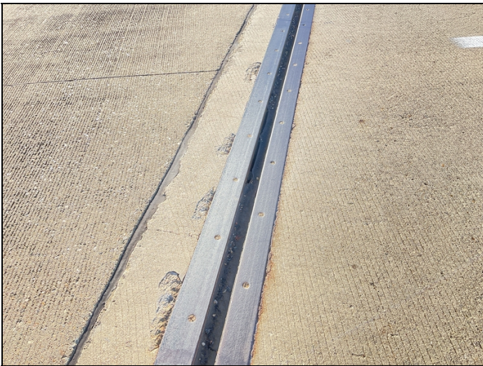
3' of joint material damage at beginning of bridge
