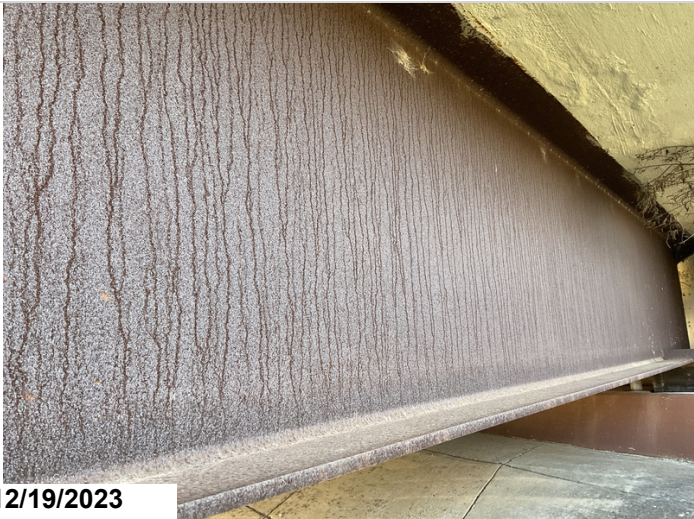
Continuous weathering steel beams
