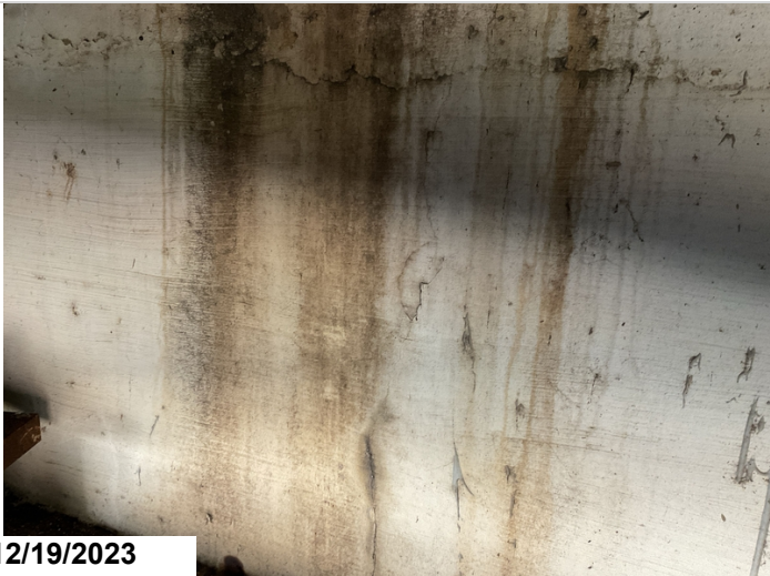
Bent 1 abutment cracking
