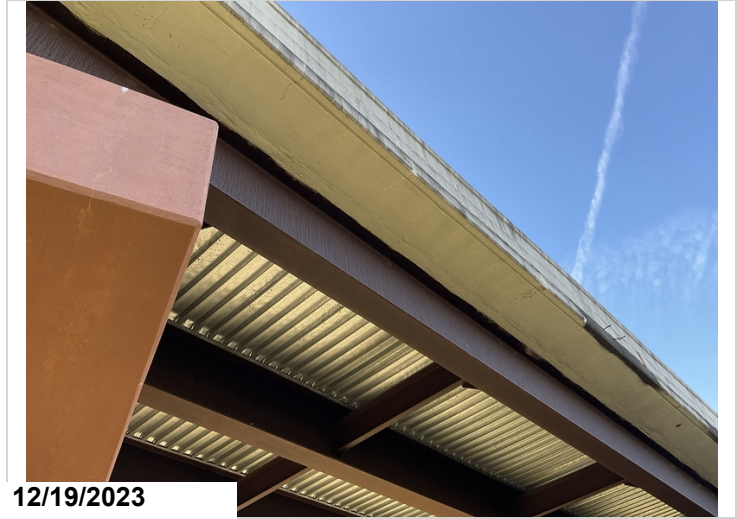
Cracking with efflorescence in deck overhangs
