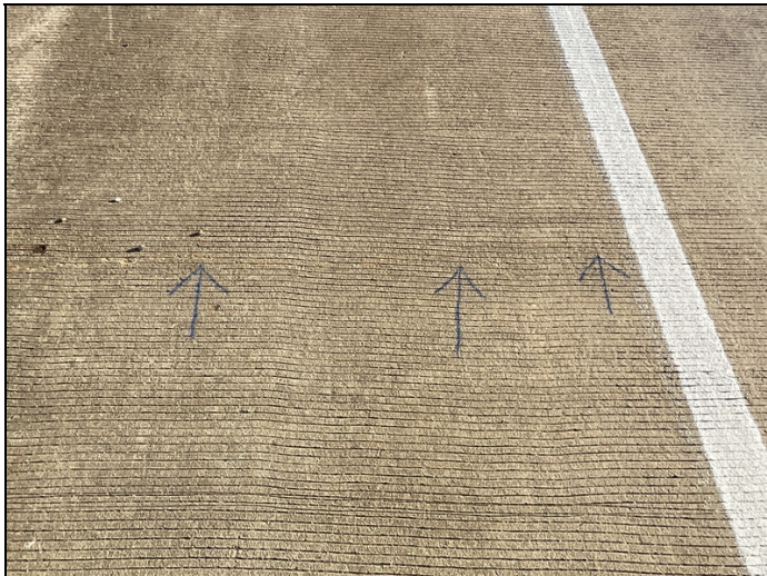
Deck cracking in various locations of deck
