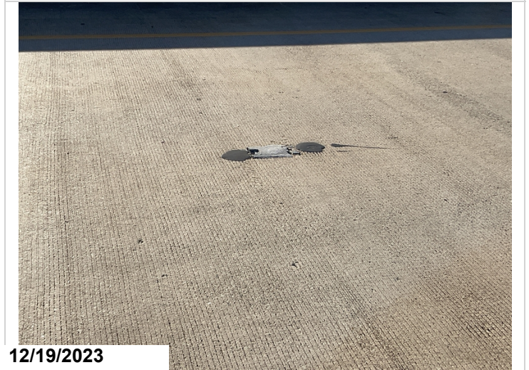
Deck patching from previous RPM removal
