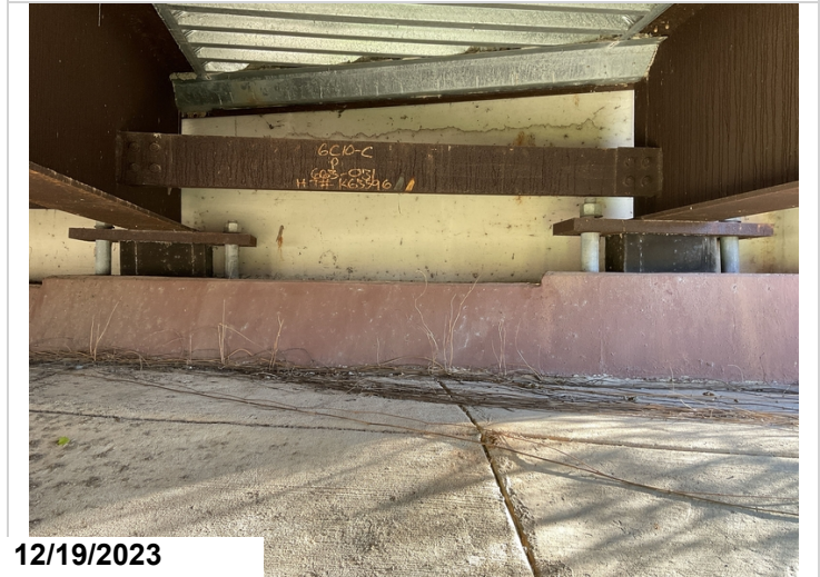
Bent 2 elastomeric bearings 1 and 2
