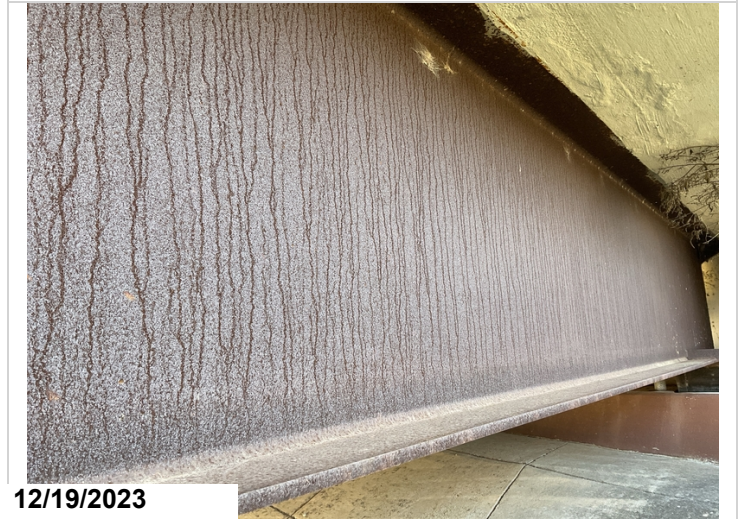
Continuous weathering steel beams
